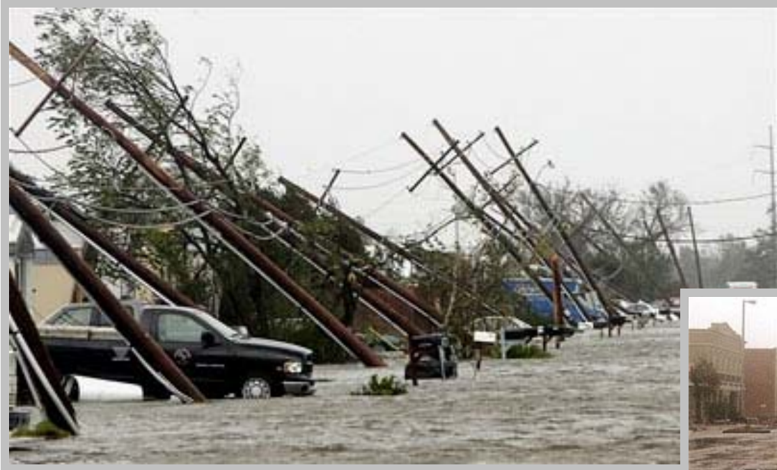
Electricity poles nearly pushed to the ground by Hurricane Katrina
