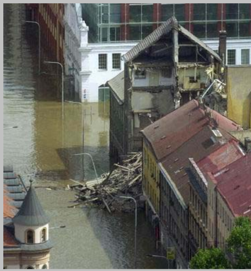
A multi-story building collapsed because of floods
